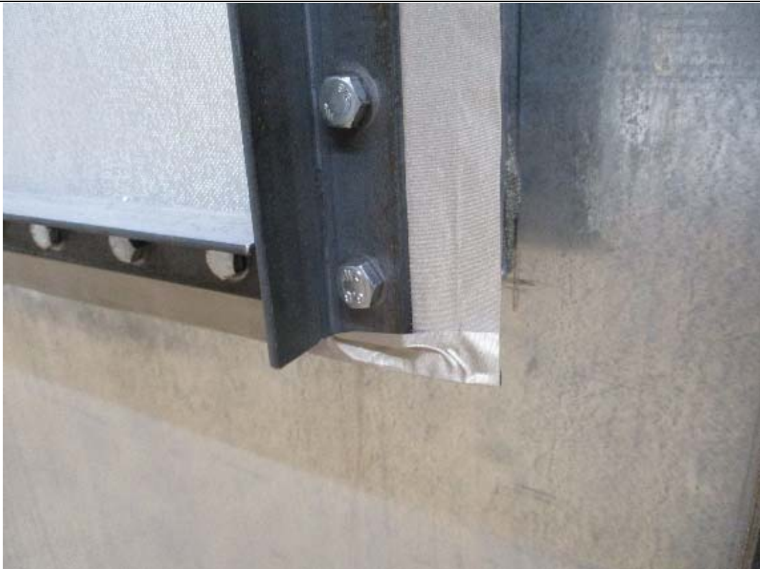
The connection between the layers was ensured with electrically conductive adhesive tape
